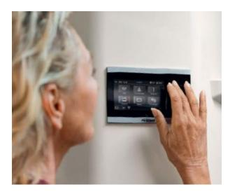
O1 Central operating unit with touch pad for monitoring and controlling the heater, water supply and batteries.
